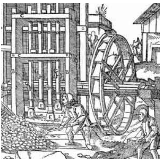
Stamping machine and waterwheel © Historic Environment Record, Cornwall Council
