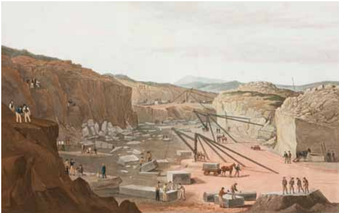
Granite obtained from quarries like Hay Tor was used as a local building material © Science Museum / Science & Society Picture Library
